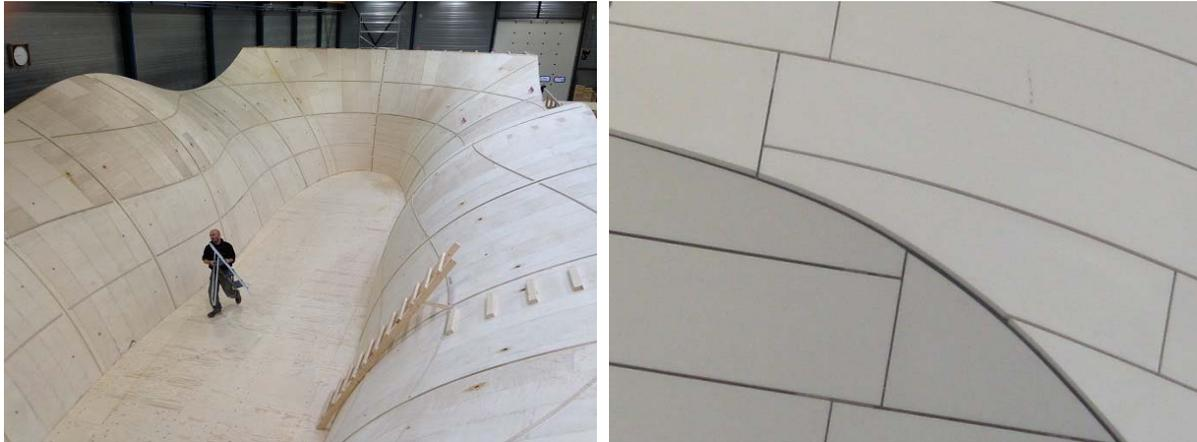
Figure 1 — Left: an example of timber formwork for double-curved bridge parts for the Verlengde Waalbrug Nijmegen, The Netherlands (Architectenbureau Zwartz & Jansma, formwork by [Verhoeven Timmerfabriek](#)), Right: concrete cladding detail of Louis Vuitton Fondation pour la Création, Paris (Frank Gehry Architects)
