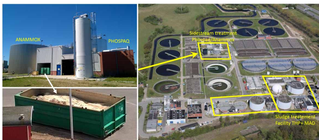
Figure 1 | Pictures of sidestream treatment plant comprising Phospaqa and Anammox reactor and the sludge treatment facility comprising THP and MAD at the centralised sludge treatment plant at Tilburg (derived from Driessen et al. 2018b).
