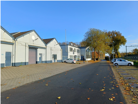
(c) Southeast buildings
