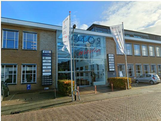
(b) Rotor building (East area)
