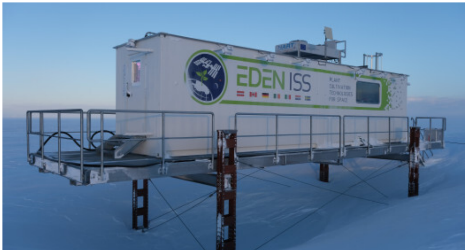
Figure 1.1: EDEN ISS Mobile Test Facility (MTF), a previous DLR Bremen project demonstrating controlled environment crop production as part of bioregenerative life support systems (BLSS). The facility was deployed near Neumayer III Station in Antarctica for a three year campaign and produced more than 1000 kg of fresh crops for the station crew. Source: [7].
