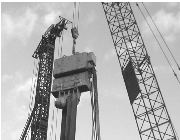
Figure 2.2 Sheet pile and vibrator
