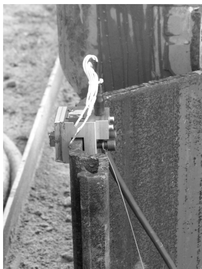
Figure 7.8 Vibration transducers at top of Z-profile
