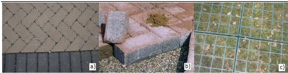
Figure 4-2(a) Impermeable Concrete PICP; (b) Porous Concrete PICPs; (c) Grass-filled PICPs.
