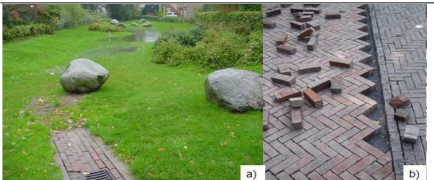
Figure 1-4 a) Bioretention swale after rainstorm, b) permeable pavement.
