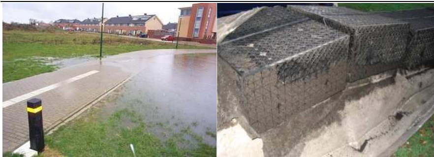
Figure 1-3 insufficient hydraulic capacity of a swale (left) and clogged infiltration system.
