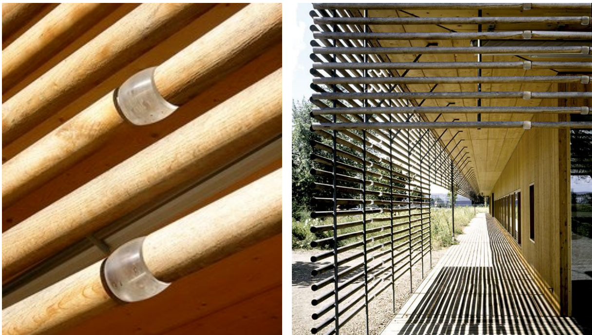
Figure 31. Craftmanship details of wooden screens.
