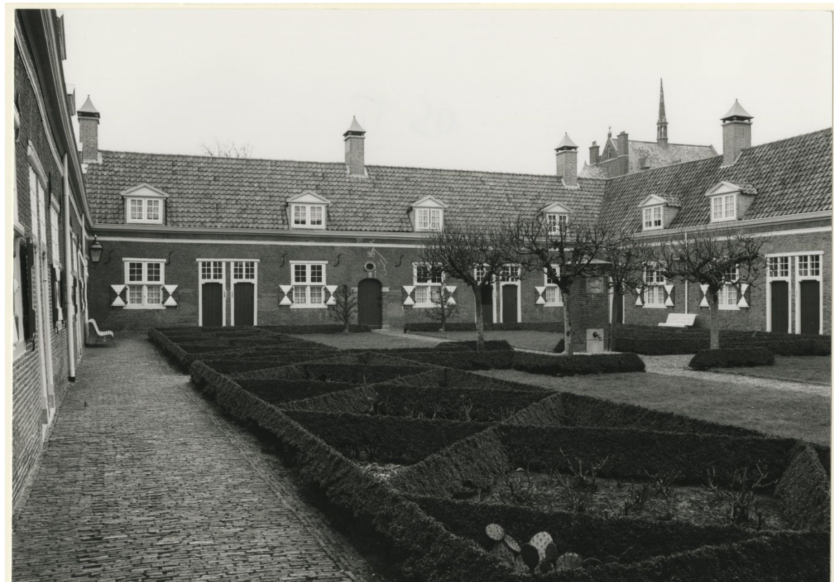
Figure 23 View of the courtyard.
