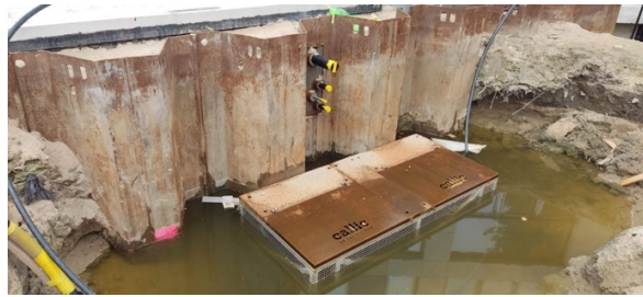
Figure 14: Inlet of a TEO-system integrated in a quay wall (H. Biemond, personal communication, October 3, 2023)
