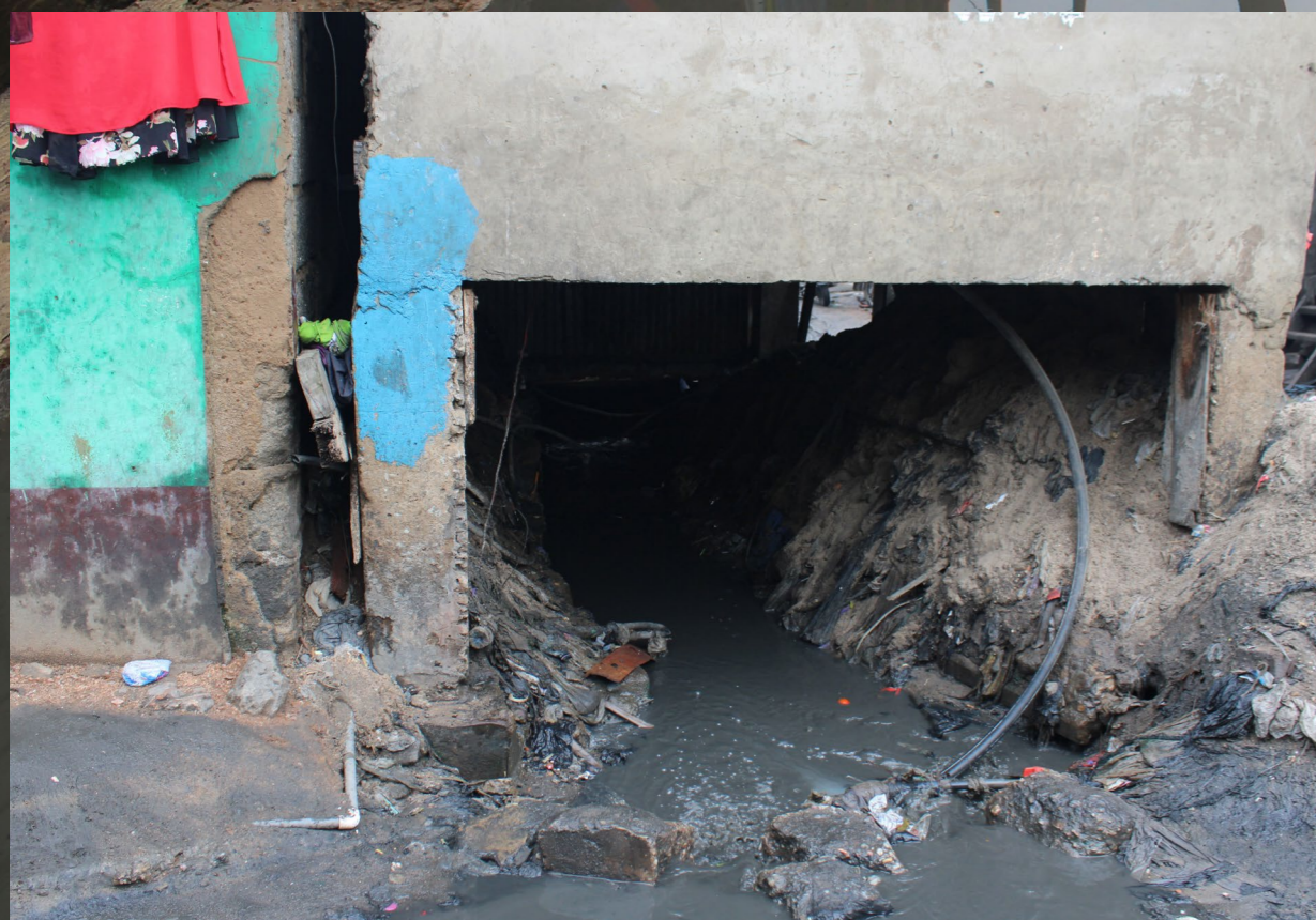
Figure 3.3 Flooding from rainfall has slashed away a dwellings foundation in Old Fadama (Photo by Author)
