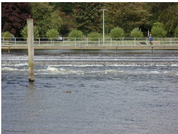
Figure 6.3 Hambleden Weir, where remedial works ruined a good canoeing spot
