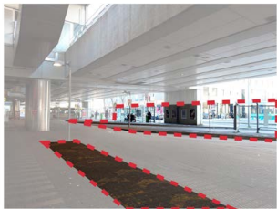
Faded wayfinding elements
