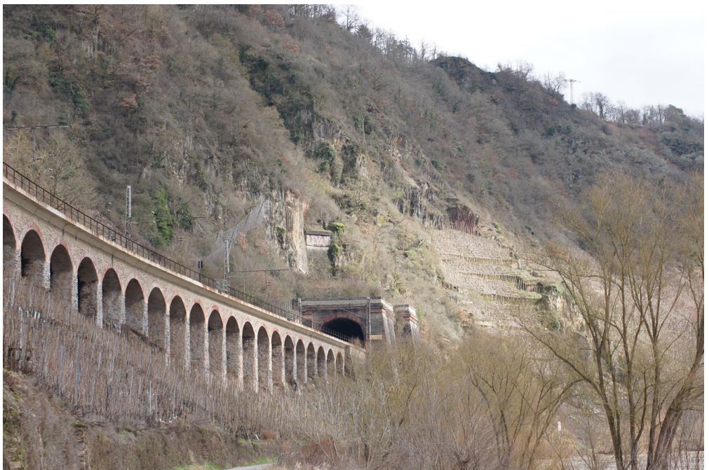
Fig. 11: The slope viaduct is iconic in the landscape of Zeller Hamm.
