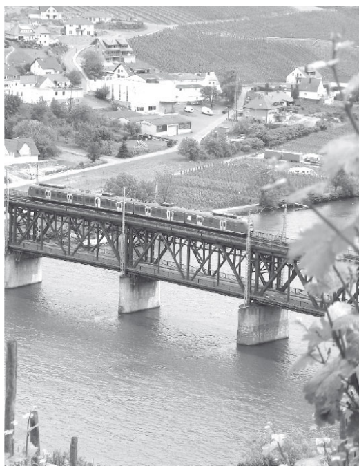
Fig. 10: Bullay railway bridge, the train crosses on the top while cars use the bottom lane.
