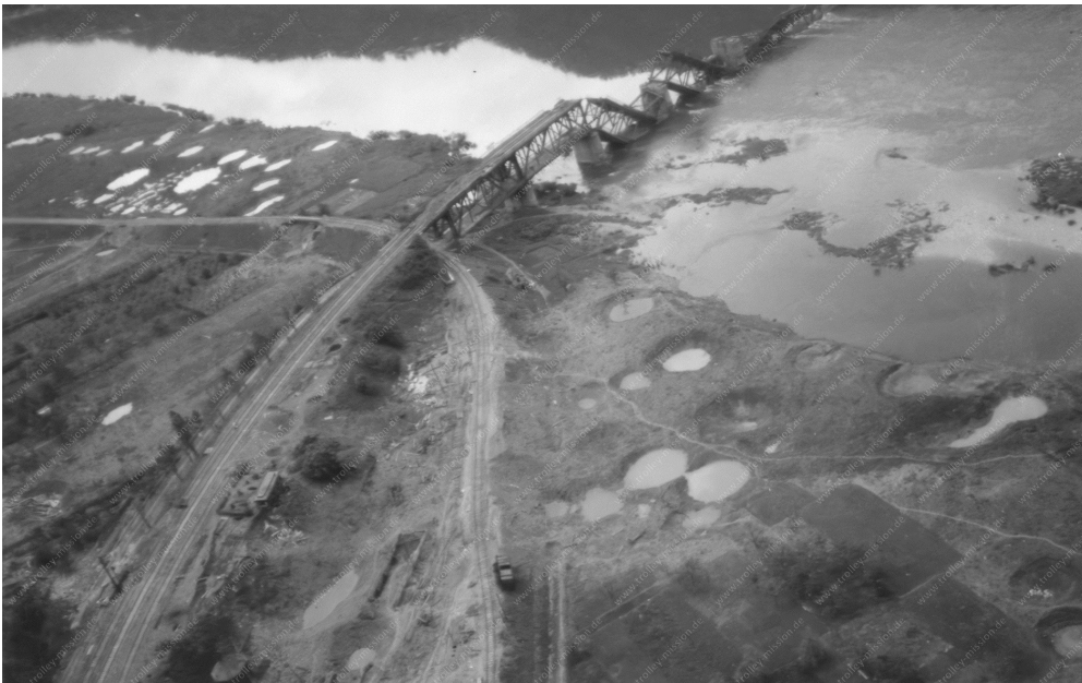
Fig. 12: Doppelstockbrücke Bullay in 1945 after bombings.
