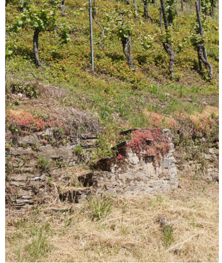
Fig. 83: Traditional drywall stairs.
