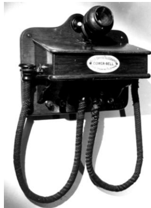
Figure 127: British Gower-Bell Telephone as used by the Post Office (1881).
