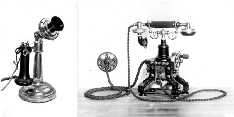
Figure 105: Candlestick Telephones by the Augusta Electric Company (1899, left), and Ericsson’s Skeleton Telephone (1892, right).
