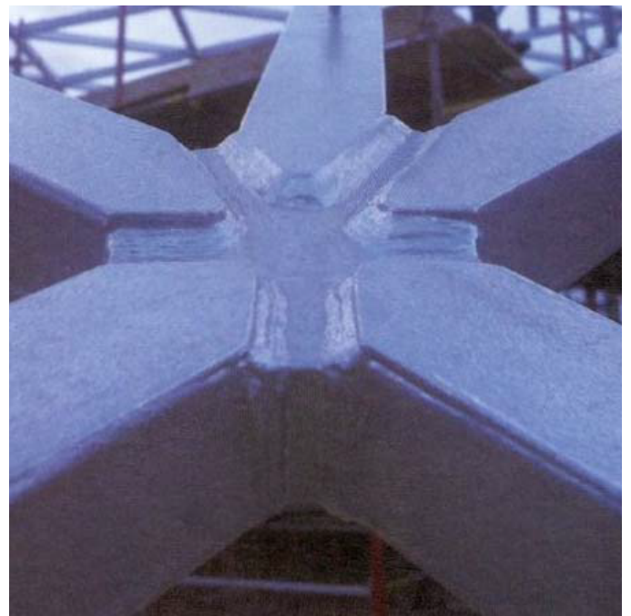
Figure 2.5.20: End-Face Connector WABI-1 at British Museum Source: Stephan et. al, 2004
