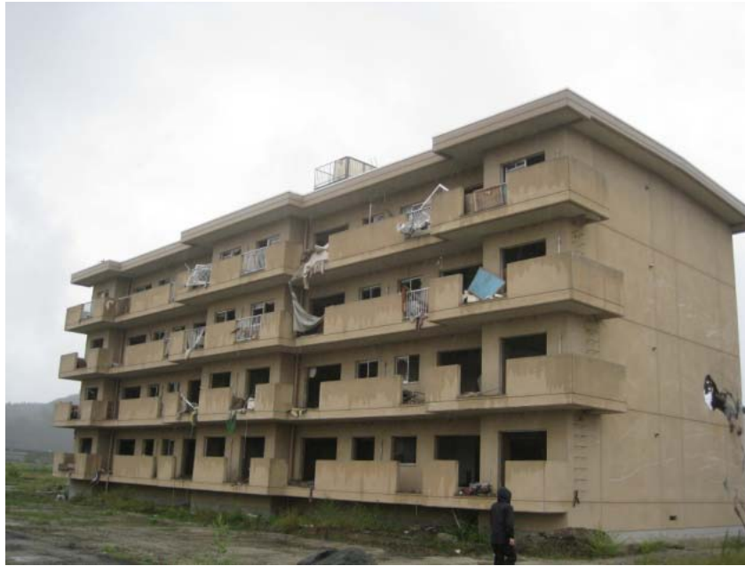
Figure 3.14: Concrete building that was overtopped
