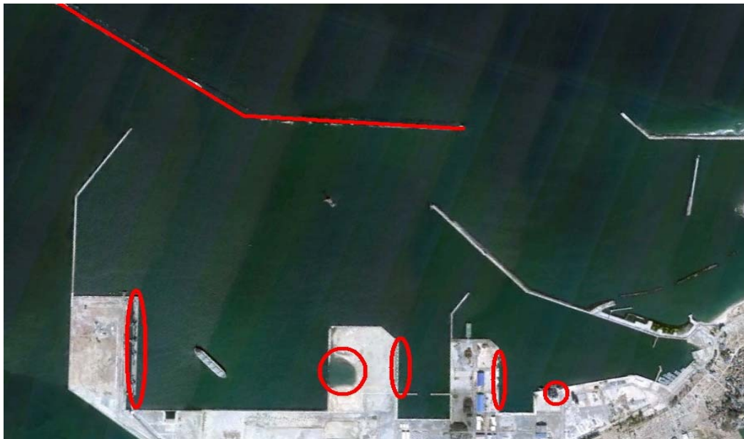
Figure 3.29: Port of Soma after the tsunami. The most severely damaged parts are indicated (Google Earth caption, 2011)
