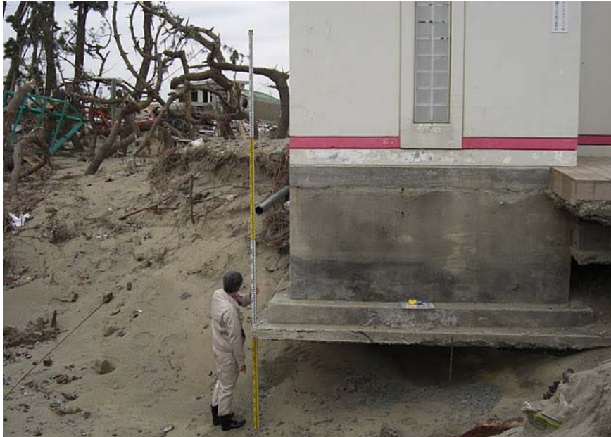
Figure 3.24: Scouring on the toe of concrete building (Source: The 2011 Tohoku Earthquake Tsunami Joint Survey Group; www.coastal.jp/tsunami2011 )
