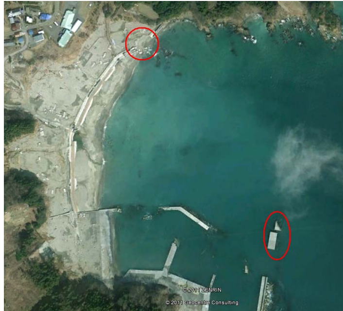
Figure 3.9: Zoom in the bay where the visited tsunami wall is located (region B). A large section of the tsunami protection dyke was broken at its north end, and severe damage of the caisson breakwater was also noted (Google Earth caption, 2011)
