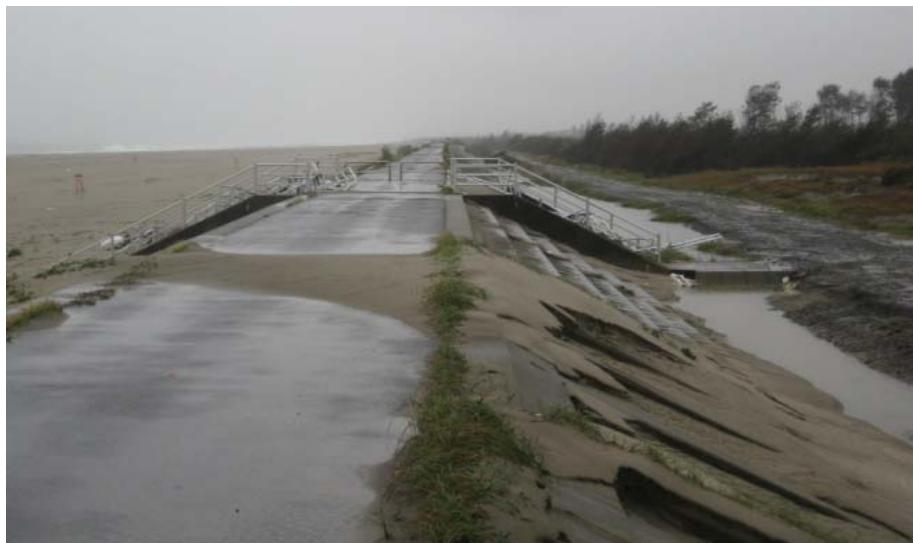
Figure 3.23: Sandy beach and sea dike at Arahama Wakabayashi-Ward
