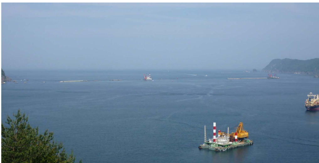
Figure 6.4: World's deepest breakwater in Kamaishi, photographed in June 2012, during its reparation
