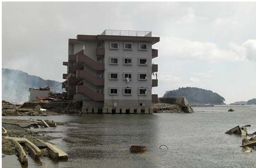
Figure 4.10: Evacuation building on the frontage that was just overtopped, people sheltered on the top of it survived (Source: The 2011 Tohoku Earthquake Tsunami Joint Survey Group; www.coastal.jp/tsunami2011 )
