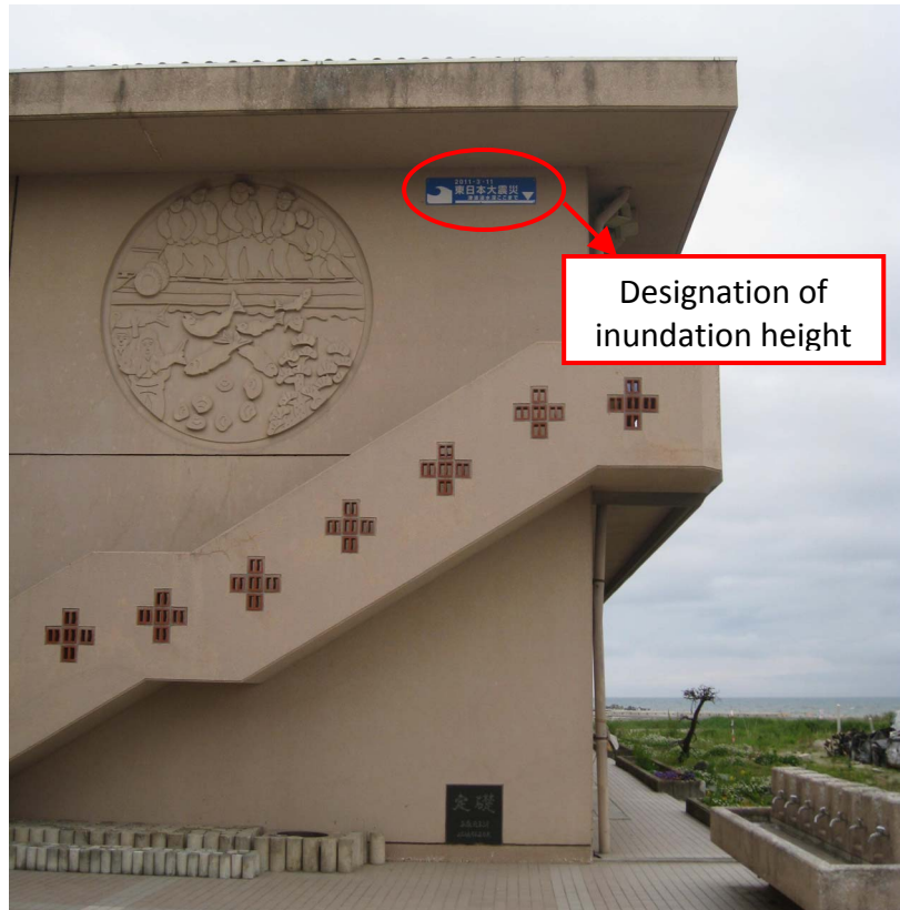
Figure 3.25: Designation of inundation height on the school building photographed in June 2012.
