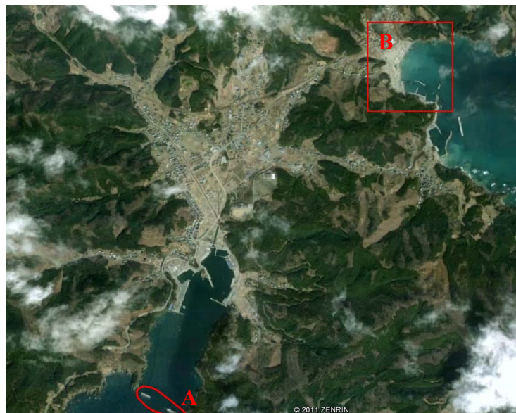
Figure 3.8: Ryori bay after the tsunami. The severely damaged caisson breakwater (A) and the sandy beach with the tsunami wall (B) are designated (Google earth caption, 2011)
