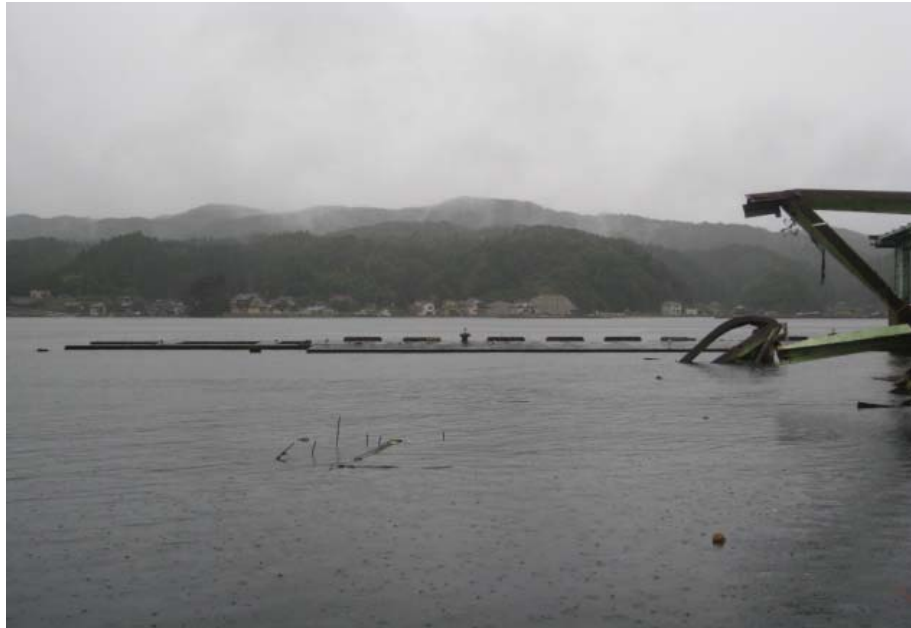
Figure 3.17: Submerged quay wall
