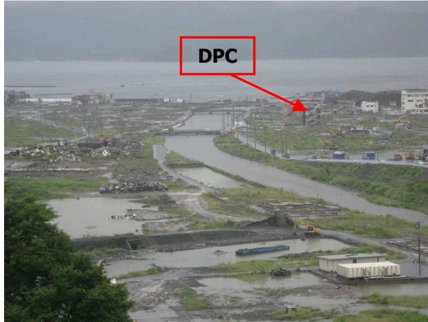
Figure 4.8: Location of the Disaster Prevention Centre of Minamisanriku
