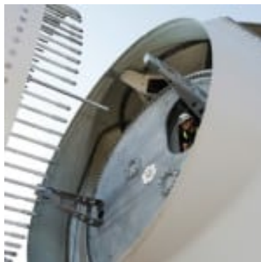
Figure 2.3: Offshore Wind Turbine Blade-Rotor Connection
