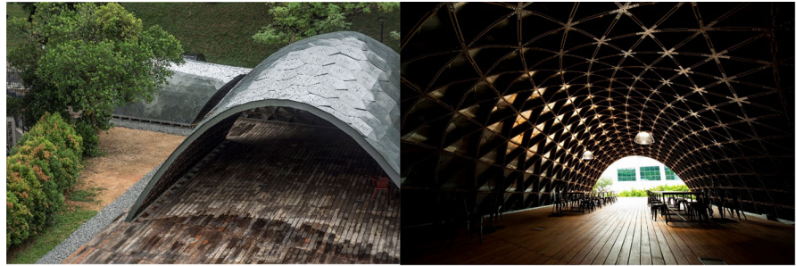
Fig. 5 Left: impression of the SUTD grid shell pavilion. Right: the mesh pattern used for the glass structure can be seen. Image source: A. Sevtsuk
