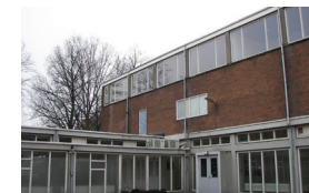
Img 69a: Inner facade west and north volume Source: author
