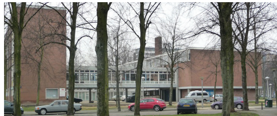
Source: I. Thoen 2013 Image of the Daniel Goedkoopschool. View to the entrance and the inner courtyard
