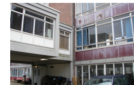
Img 69b: Inner facade south and east volume Source: author
