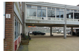
Img 69: East facades Source: author
