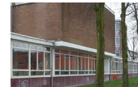
Img 68: West facades Source: author
