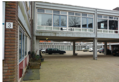
Img 77: Building part 4, east volume Source: author
