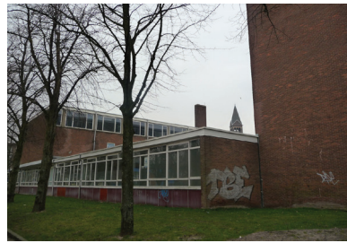
Img 75: Building part 2, west volume Source: author
