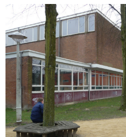
Img 78: Building part 5, west volume Source: author
