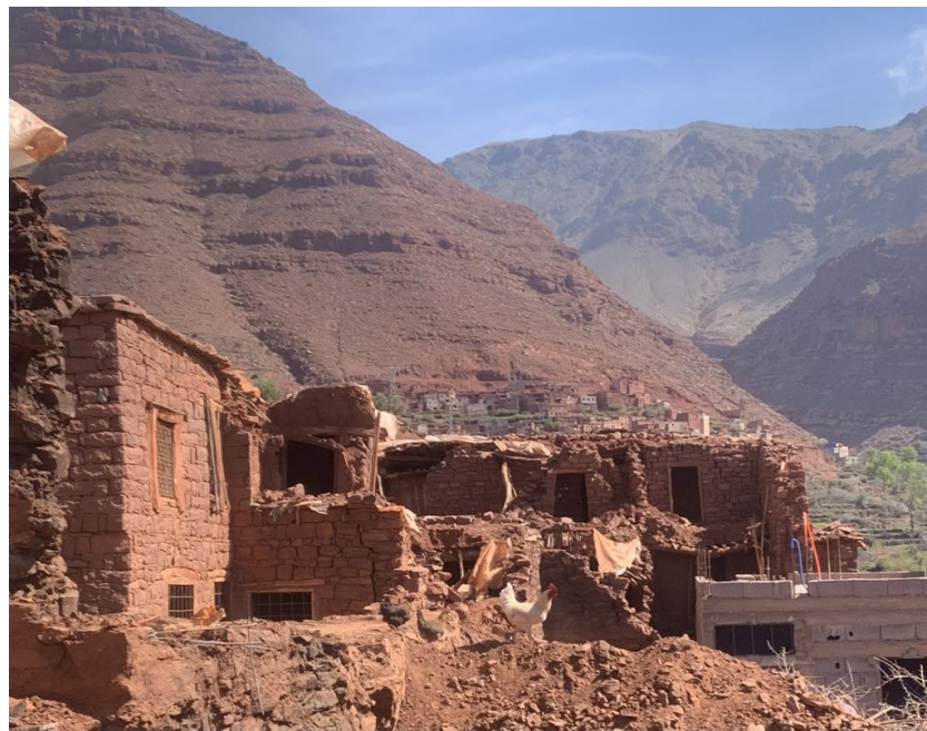
(c) First-hand photograph taken in the El Haoz region of Morocco, approximately 5 months after the 2023 Marrakesh-Safi 6.9M earthquake. Uniquely, residences were interdependent to each other as the lack of centralised planning policies allowed different families to expand on existing residences organically, making the financing of repairs challenging.
