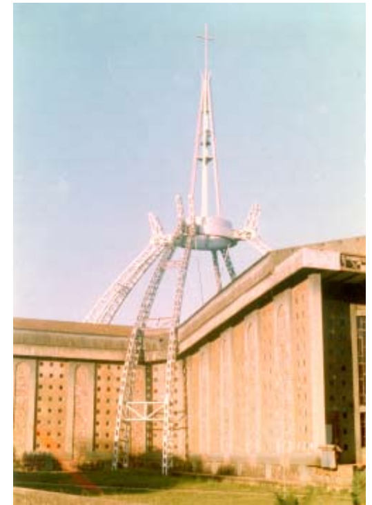
The Mater Misericordia in 1991. The covering of the flying buttresses has completely disappeared and the roof is in a bad state.
