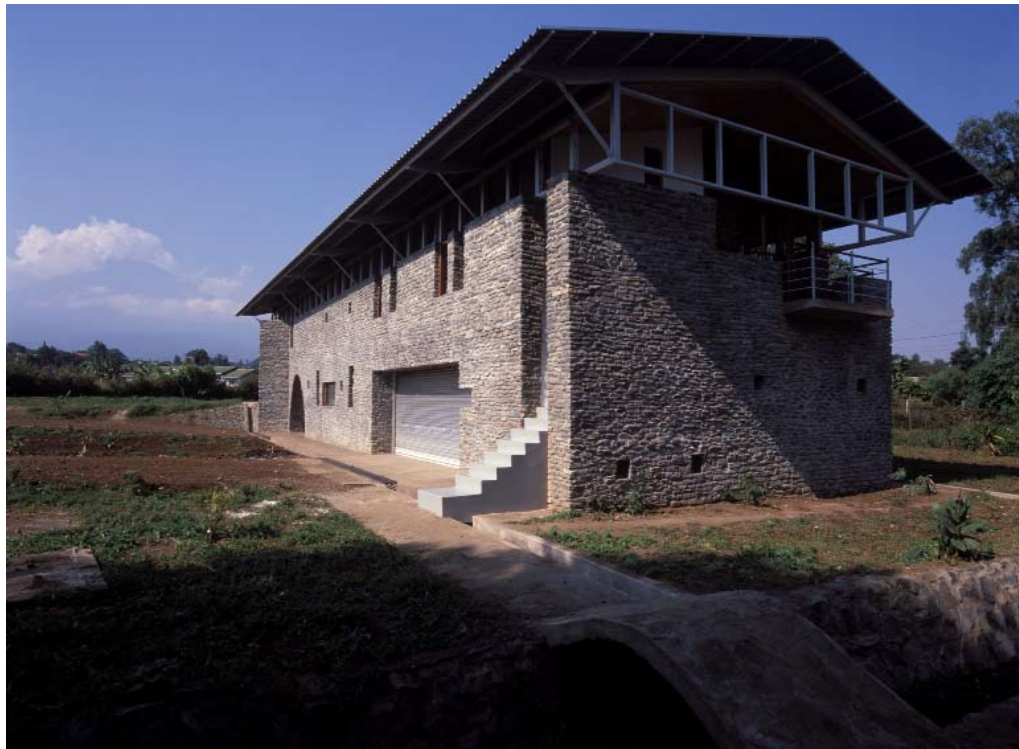
Van der Wel House in Arusha. The house is earthquake-resistant and built of locally obtained limestone with 60 cm thick walls and an cantilevered Vierendeel-girder serving simultaneously as a continuous band of clerestory windows. [See also p. 206] Photo: Nick Parfitt
