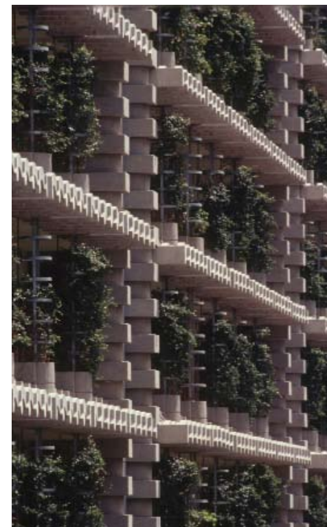
Eastgate building in Harare by Mick Pearce. This great office block uses half the energy of a conventional building because of the ingenious ventilation system that was inspired by a termite-heap. Photos: David Brazier
