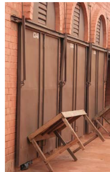
The steel, up-and-over doors-cum-awnings of the market of Koudougou. Photo: Belinda van Buiten
