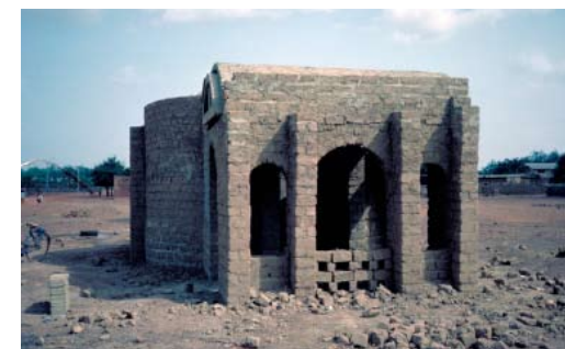
The completed structural shell of the DGUT field office.
