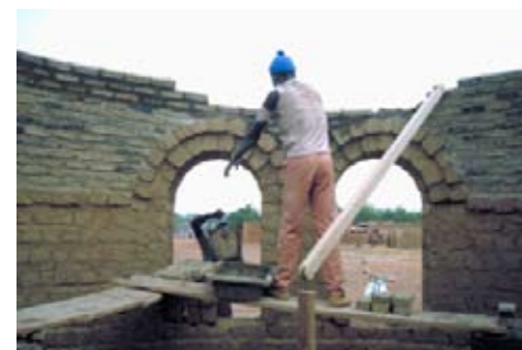
The construction of the DGUT cupola without use of forms.
