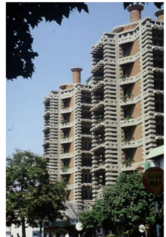
Eastgate building in Harare by Mick Pearce. This great office block uses half the energy of a conventional building because of the ingenious ventilation system that was inspired by a termite-heap. Photos: David Brazier
