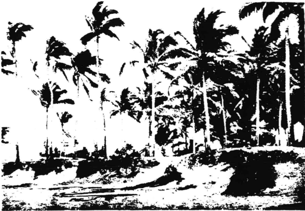
Plate F.6 (a) Coastal erosion of sandy beach at Miramar, Goa.
