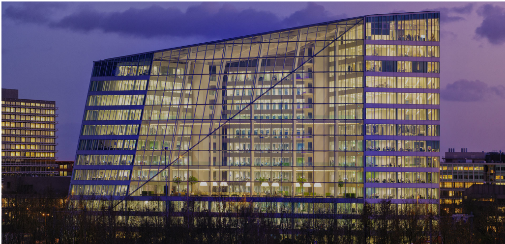
Figure 50 - The Edge 'Most sustainable and smartest office in the world' (OVG Real Estate)
