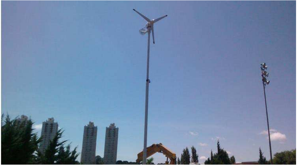
Figure 10. Final aspect of Wind Turbine Installed
