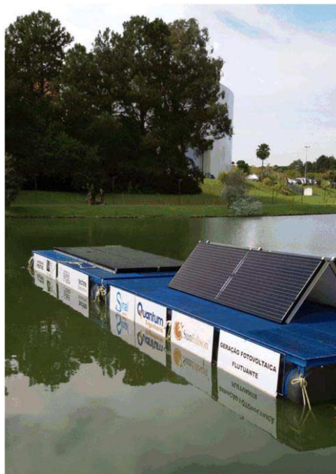
Figure 4. Ferry Solar Photovoltaic Panels Details
