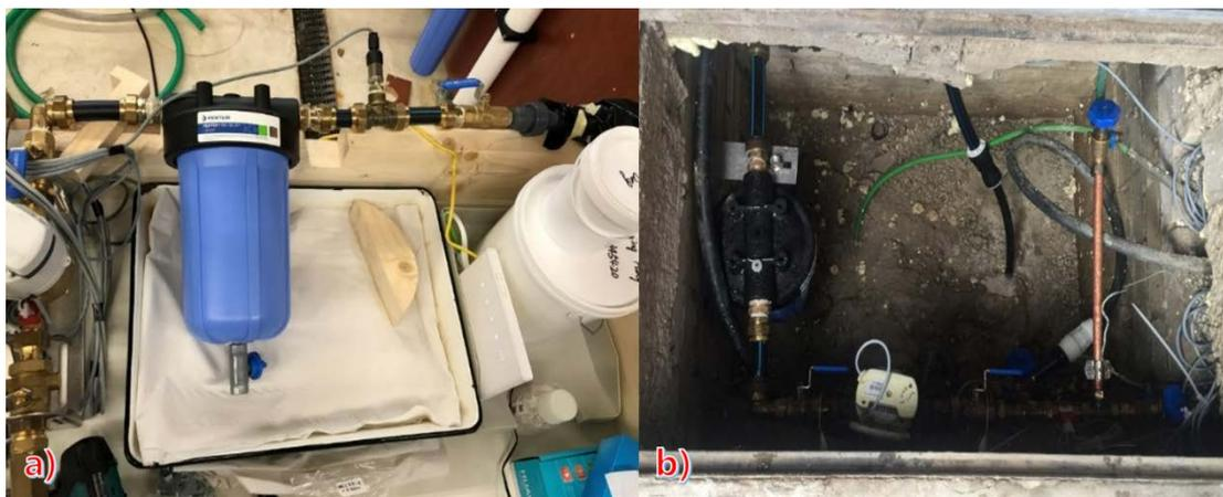
Figure 2.3 a) Smart Water Meter set-up; b) Smart Water Meter was installed in the ambient in a household
