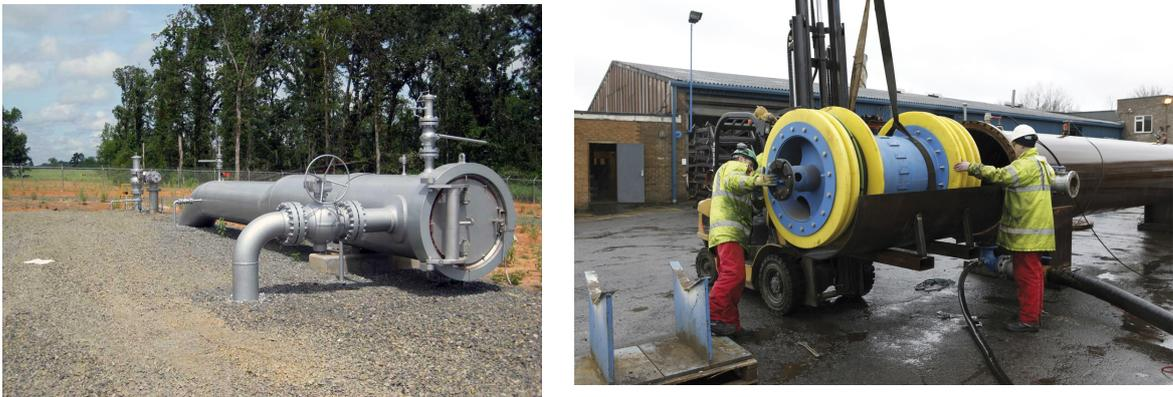
Figure C.2: **Left:** A pig launcher for a gas pipeline. **Right:** A pig being inserted into a pig launcher. The yellow plastic disks seal against the inside of the pipe to propel the device and to remove loose sedimentation or scale buildup [130]
