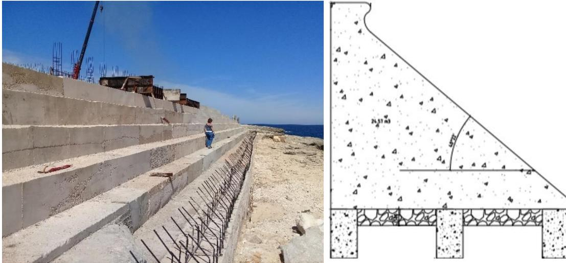
Figure 6 – Current defense wall under construction & Current defense wall design
