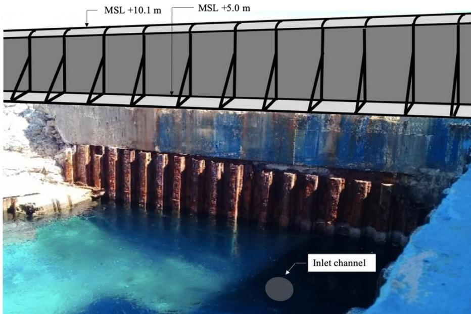
Figure 175 - Visualisation of the sea defense on top of the inlet structure
