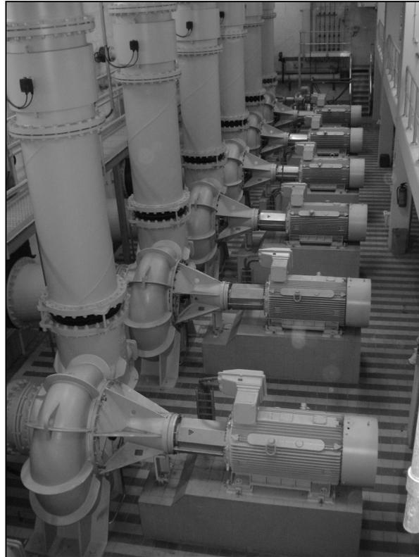
**Figure 4-2:** Influent pumps at the influent pumping station of wwtp Eindhoven. On top, the electromagnetic flow sensors in separate flanges build into the discharge lines of the pumps.
