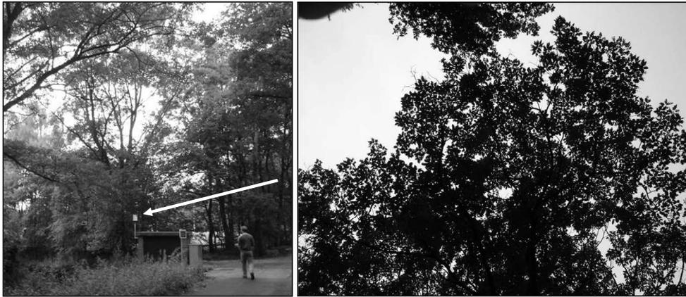
**Figure 3-5:** Incorrectly installed tipping-bucket raingauge in Sterksel. The left picture gives a situation overview showing the raingauge attached to a small pumping station; the picture on the right gives the view upwards as seen from the sensor.
