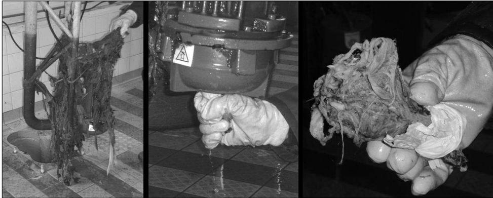
**Figure G-3:** (left picture) pollution around a by-pass pump as observed directly after the truss construction has been lifted from the wastewater; (middle picture) the suction mouth of the pump obstructed by a ball of tissue material and other coarse materials; (right picture) the obstruction after removal from the suction mouth
