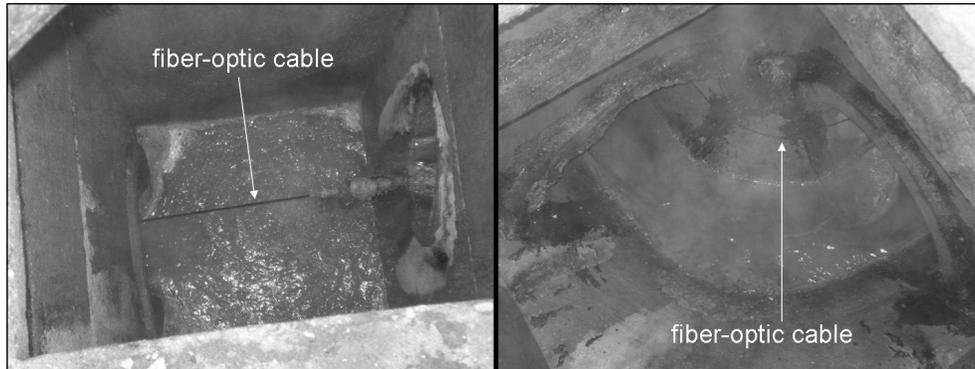
**Figure 7-20:** Locations where the fiber-optic cable is just above wastewater level due to an invert level difference (left picture) and due to the cable being pulled too taut around a sharp bend (right picture).
