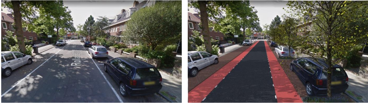
Figure 6.5: Rollandslaan before (l) and after (r) the application of asphalt collectors (Own ill. based on Google Maps)
