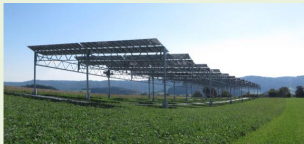
Figure 5.13: Combined agriculture and solar panels ( www.ise.fraunhofer.de )
