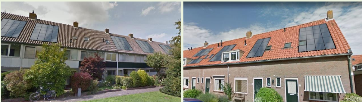
Figure 5.6: Integration of PVT-panels in Abraham Mensstraat (l) and Midden Tuindorpslaan (r) (Own ill.)
