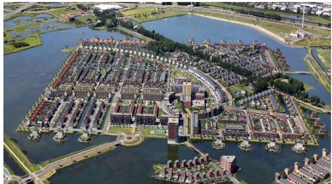
Figure 2.13: Key figures and aerial view ( heerhugowaardstadvandezon.nl , n.d.)
