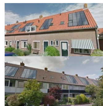
Figure 6.4: Solar panels integrated in the roof (Own ill.)
