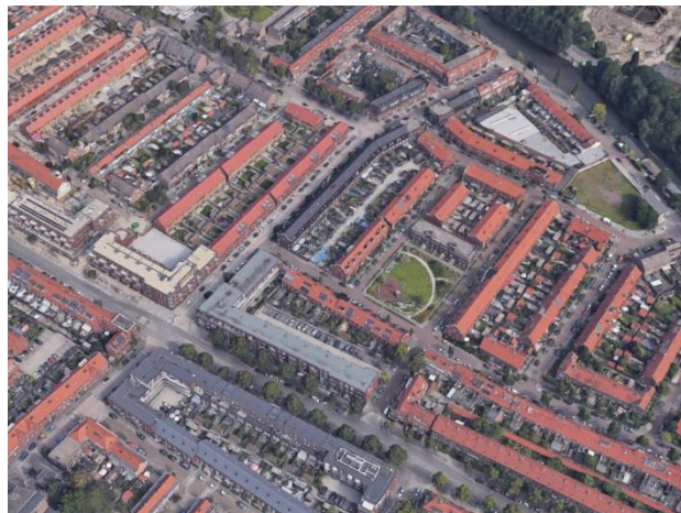
Figure 2.16: Key figures and aerial view of the neighbourhood 'Ondiep' (Google Maps)
