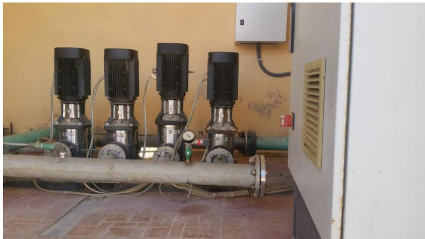
Figure C.14: Picture of the pumps for distribution of the freshwater to Blau Arenal Hotel
