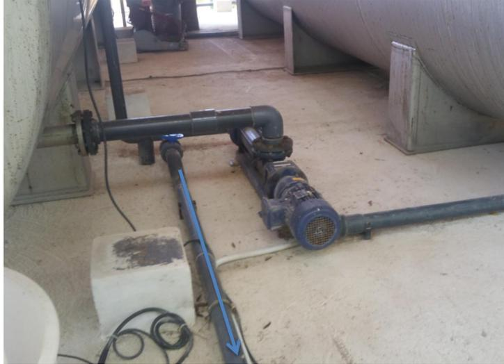
Figure C.10: Picture of the sludge pump, with direction of flow indicated
