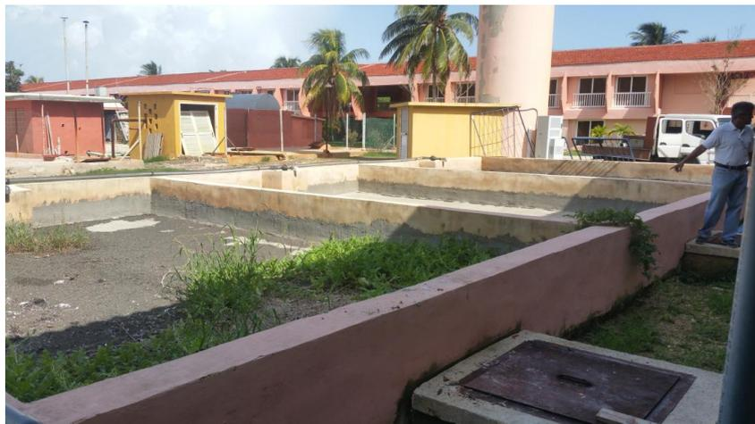
Figure C.11: Picture of the basins, where sludge naturally dries
