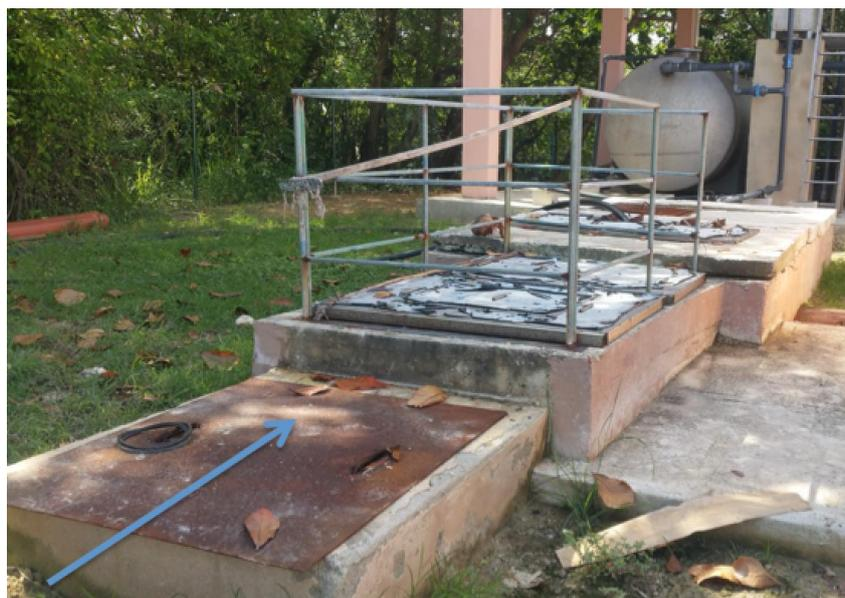
Figure C.4: Picture of underground reservoirs for untreated waste water, with direction of flow entry indicated
