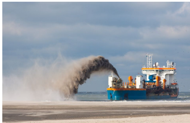
Image 8: Artificial sand replenishment to prevent coastal erosion (Ingenieur, 2025)
