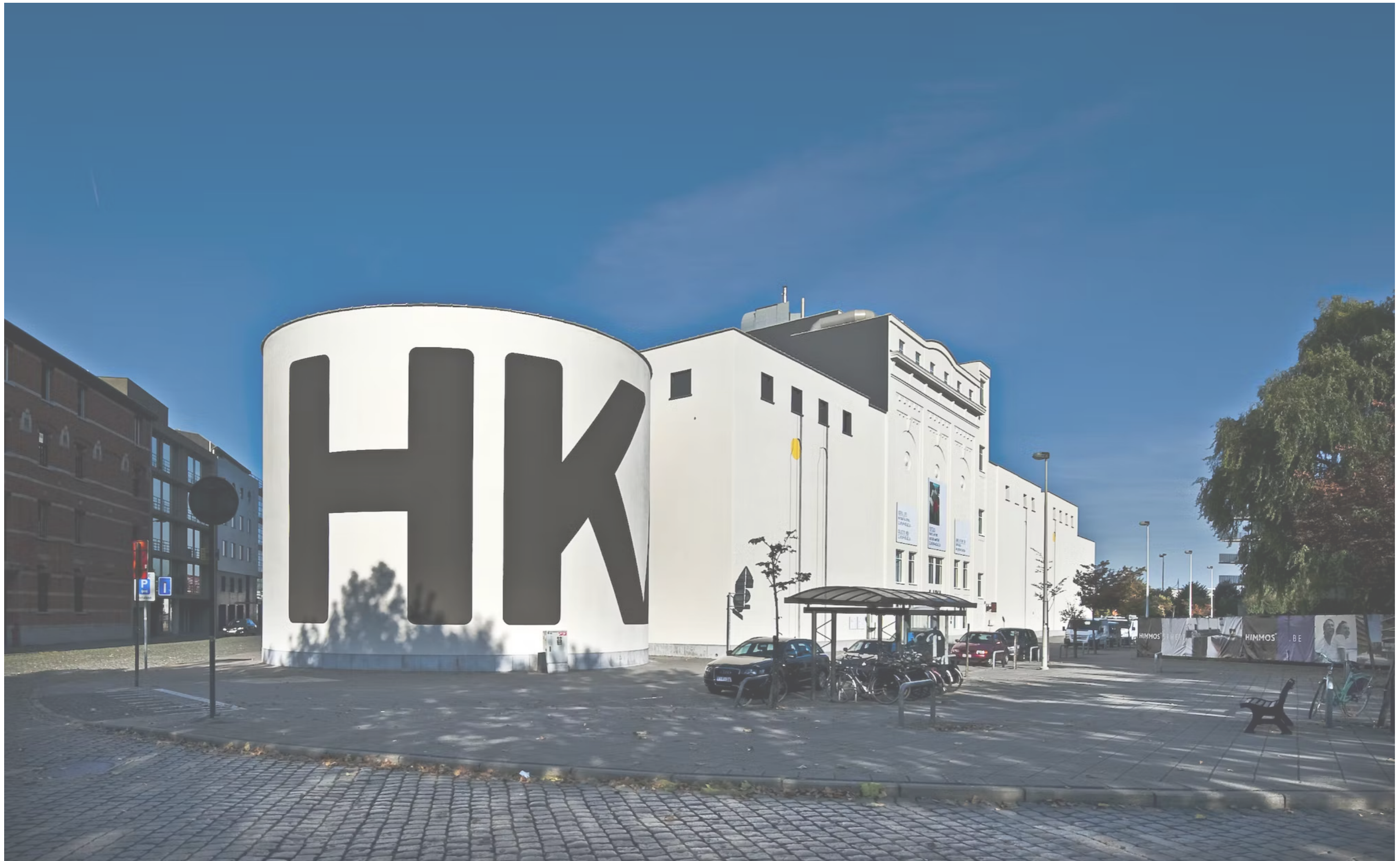
Figure 1: "Current MHKA Building", MHKA, Antwerp, Belgium, 2022
