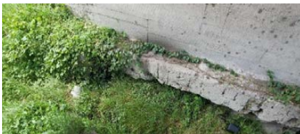
Figure 10. Bridge piers in 2024
