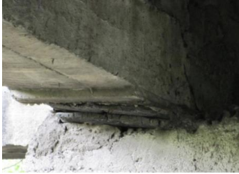
Figure 4. Wooden supports of the bridge in 2013
