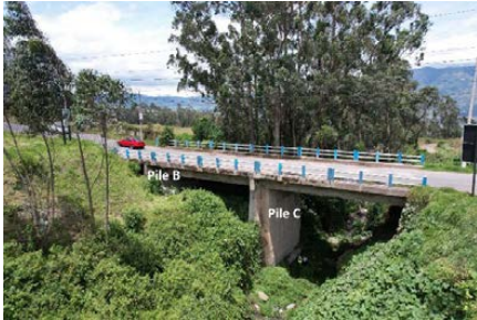
Figure 2. Bridge selected for visual inspection
