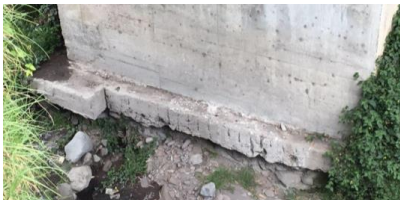
Figure 6. Piers of the bridge in 2014
