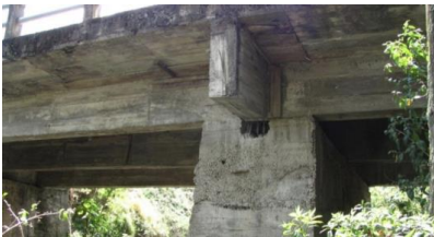
Figure 5. Piers of the bridge in 2013
