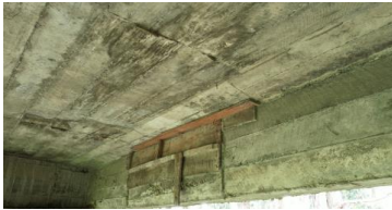
Figure 9. Beams of the bridge in 2024
