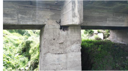
Figure 11. Bridge piers in 2024
