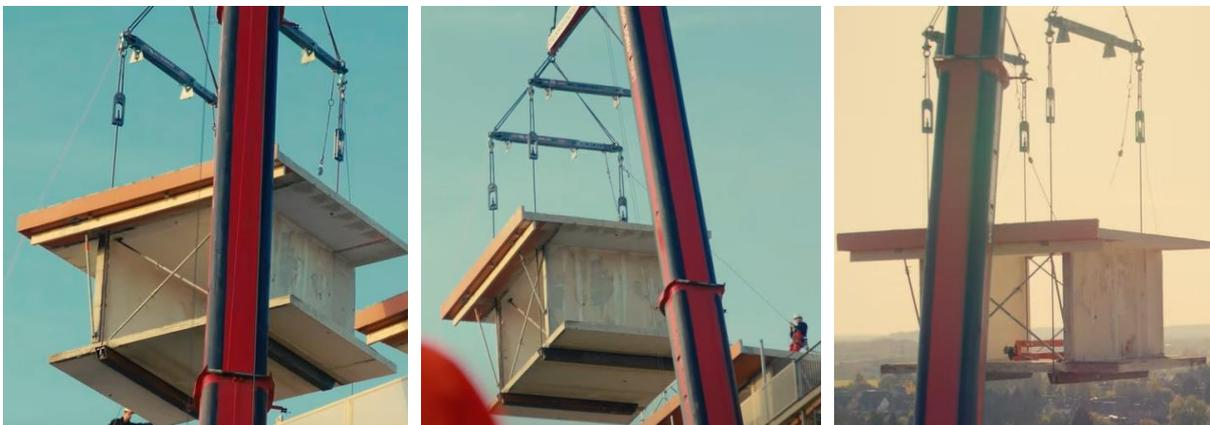
Figure 6.7: Hoisting of the in situ element (SUPERLOCAL HEEMwonen, 2021)
