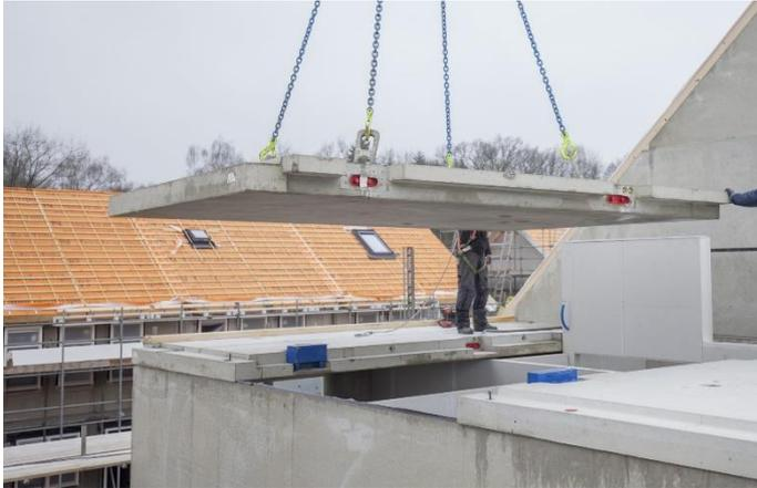
*Figure 4.9: Prefab casco floor (Eisma Content Marketing , 2018)*
