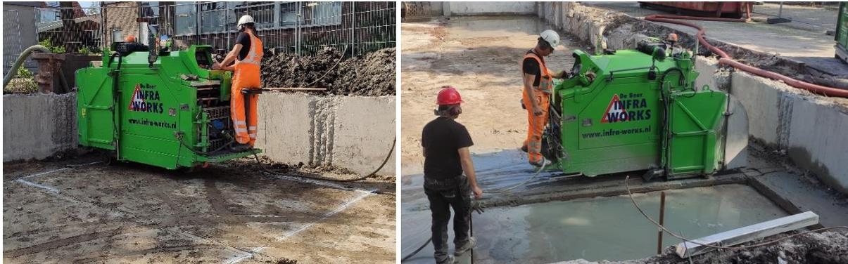
Figure 0.41: Sawing of concrete (Lenears, 2022)
