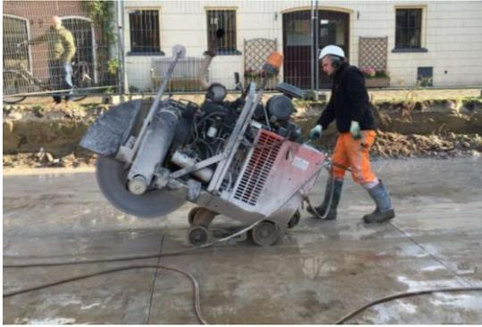
Figure 6.6: Sawing of concrete (Stelling, n.d.)
