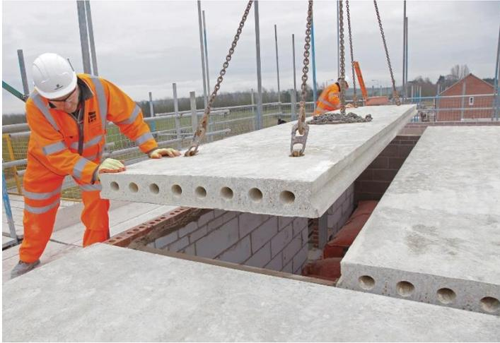
Figure 3.5: Hollow core slab element (Bison Precast, n.d.)
