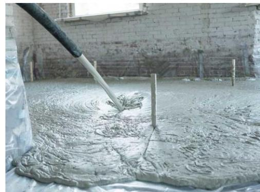
Figure 0.51: Pouring of foam concrete (Loon, 2021)
