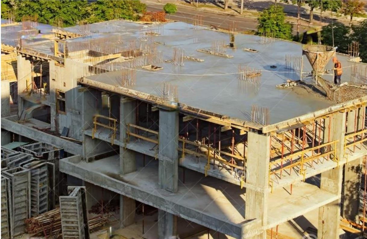
*Figure 3.2: Monolithic floor under construction (Gomeniuk, n.d.)*
