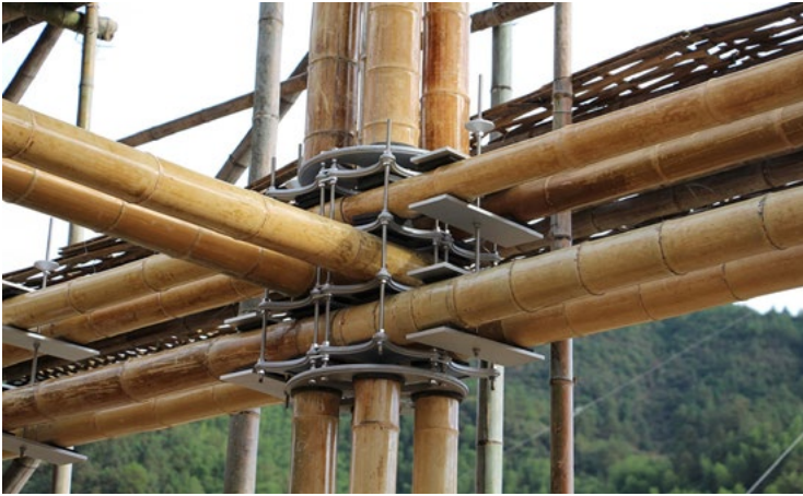
Figure 12: Connections Using natural form of Bamboo.
