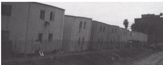
Figure 8.7. Soft story collapse (DHUD-OPDR, 1994); Relationship between the natural period of the soil and alluvial depth (Seed, 1970)
