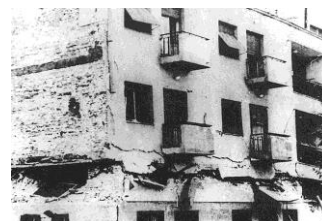
Figure 8.9. Masonry houses in the earthquake of 1976 Slovenia (Lutman et al., 2002)
