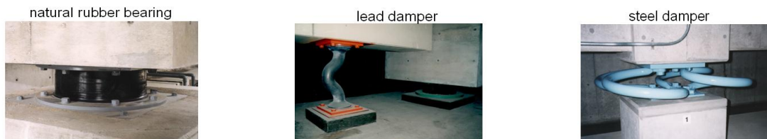
Figure 4.11. Rubber and other resilient materials and systems in foundations (photo: Saito, T.)
