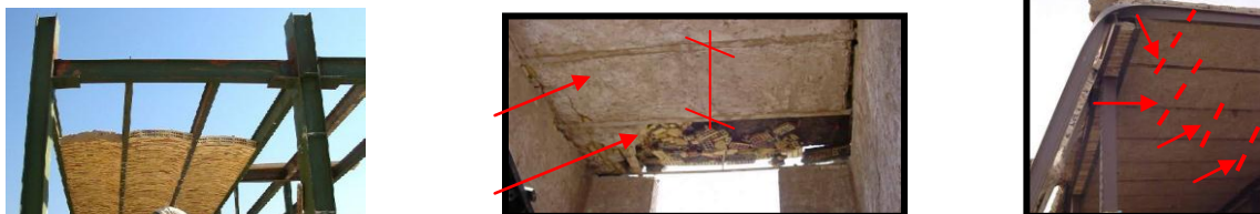
Figure 8.8. Examples of jack arch or Tagh zarbi roof system
