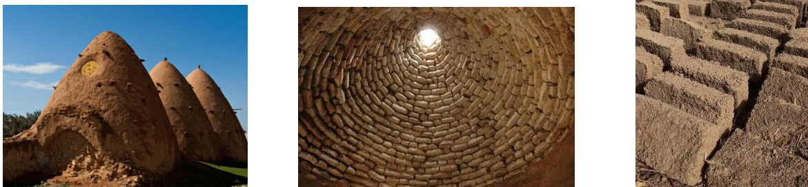
Figure 5.4, Beehive houses in Twalid Dabaghein, their high-dome's interior structure, and the applied adobe brick (source: first photo from Christopher 2009, second and third from Bikash, 2010)
