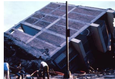
Figure 8.6. A multi-storey concrete frame structure with brick infill wall (photo: USGS, 2006).
