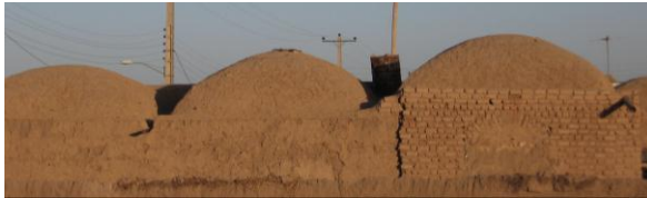
Figure 5.39. Undamaged adobe dome construction, demolition of modern materialised
