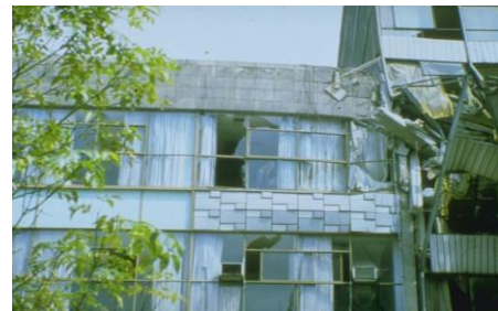
Figure 8.5. Collapse of two adjacent building with different height (source: ESDEP, 1993)
