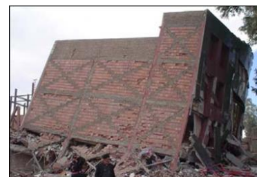
Figure 8.12. Due to instability of the soil the entire rigid structure was turned (photo: Google image)
