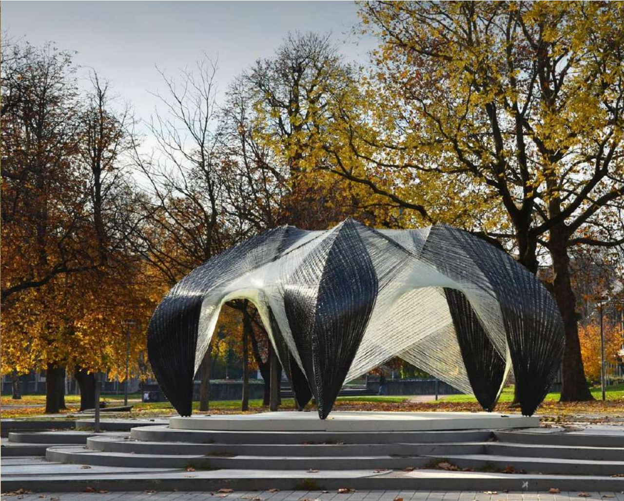
Knippers J. ICD/ITKE Research Pavilion 2012: Coreless Filament Winding Based on the Morphological Principles of an Arthropod Exoskeleton*. 2015.
