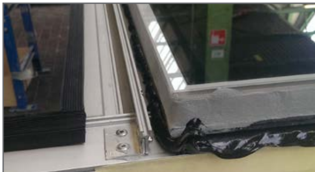
Figure 7.1.9 - Flushing of the mixer / pump and the sealant before tooling illustrate waste. (own ill.)
