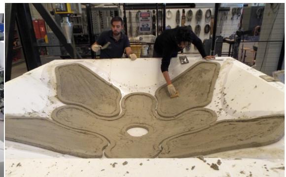
(b) Creating a double-curved shell structure using a combination of 3DCP and casting on an adaptable mould, from [7].
