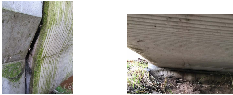
(a) Crack close to the support of the bridge due to tensile stresses in vertical direction (b) Crack at the bottom of the bridge due to tensile stresses in transverse direction
