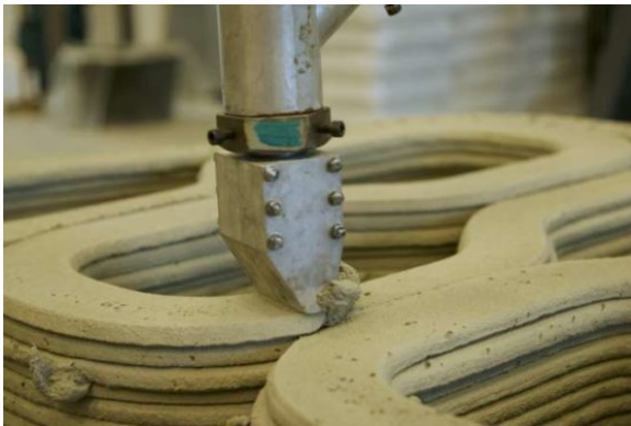
(a) Printing with a rectangular nozzle, from [11].
