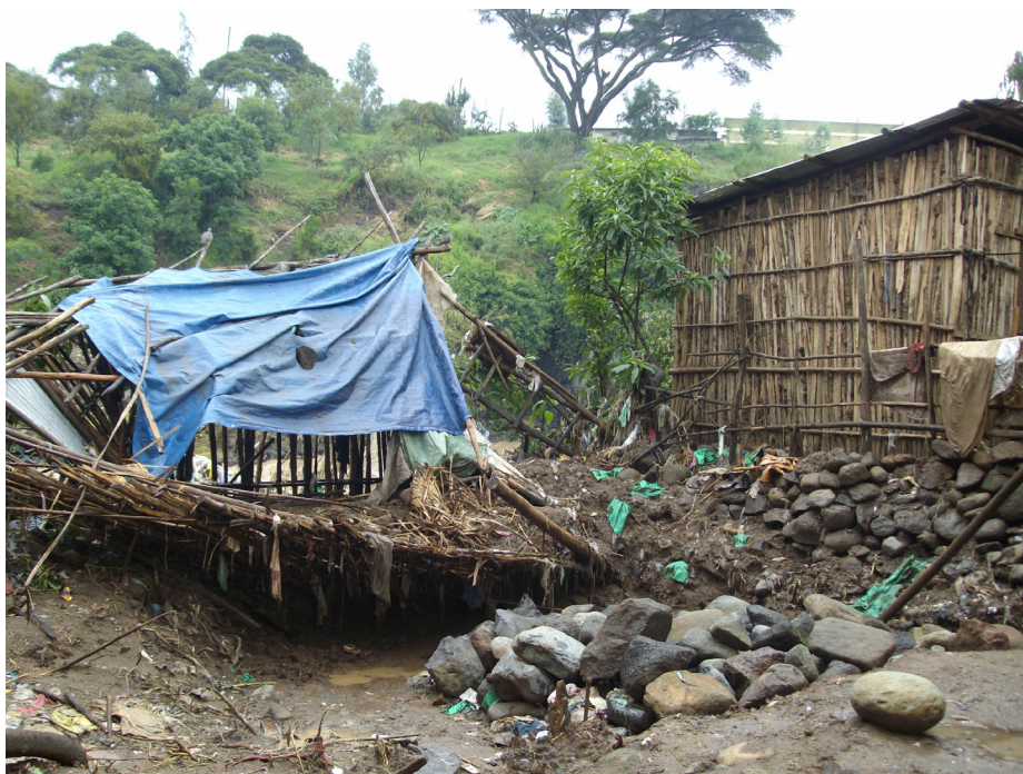
Figure 5: House that is partly washed away by flooding of the Akaki river. Photo: Franklin, M. (2008). Former house . In Flickr.
