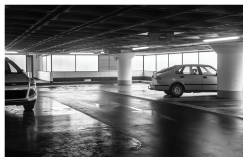
The parking garage has very low ceiling heights which makes it difficult to use the building for other functions.
