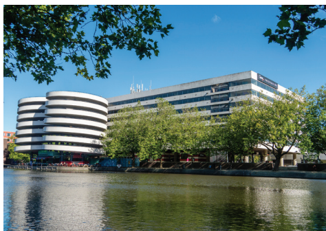
The parking garage has a striking shape seen from the Singelgracht.
