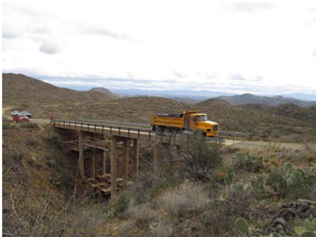
**Fig. 1.** Diagnostic load test on a rural one-lane concrete slab bridge. (Image by Jesse Grimson.)
