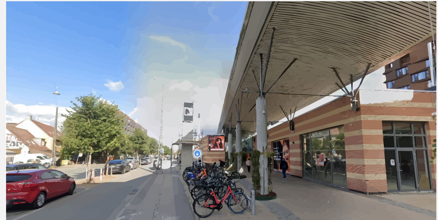
Main entrance of shopping mall
