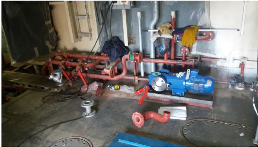
Figure 22: Installation of pipes of a ship in COTECMAR shipyard.
