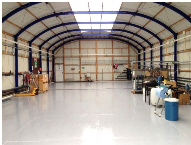
Figure 34 Delft Blue Innovations (DBI) pilot hall at the Harnaschpolder WWTP.
