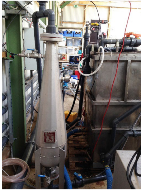
Figure 20 Speece cone at the Harnaspolder WWTP, The Netherlands (source: C. M Barreto).
