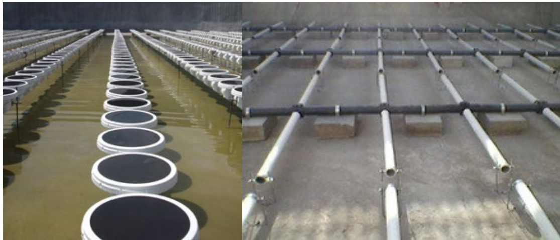
Figure 19 Disc and tubular diffusers for fine bubble aeration (Stanford Scientific International LLC).
