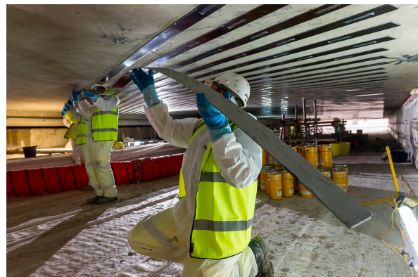
(b) Pre-cured laminates applied with an adhesive [20]
