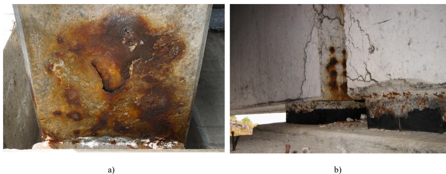
Fig. 30. Corrosion cracking in bottom of pretensioned girders: a) significant corrosion cracking in the NIB girder bottom flange near support, bridge close to Kristiansund; and b) corrosion cracking and spalling in the NIB girder-ends, photo by NPRA [7].
