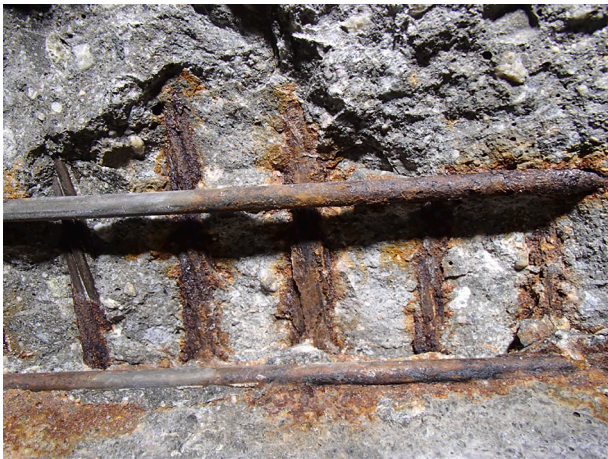
Fig. 7. Corrosion in the bottom layer of strands found near the middle support in an NIB girder in Hafstrfjord Bridge near Stavanger.
