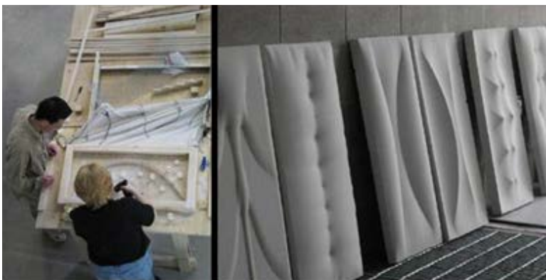
Figure 18 [top left] Fabric casting principles: Membrane is stretched across a pre-defined border into which concrete is cast source: Vergaeg, 2010
