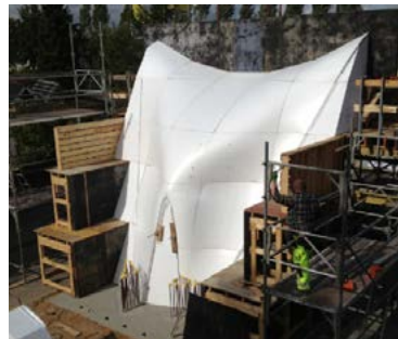
Figure 4 : Use of milled formworks on free-form concrete element - effectively building the structure twice. source: tailorcrete.com
