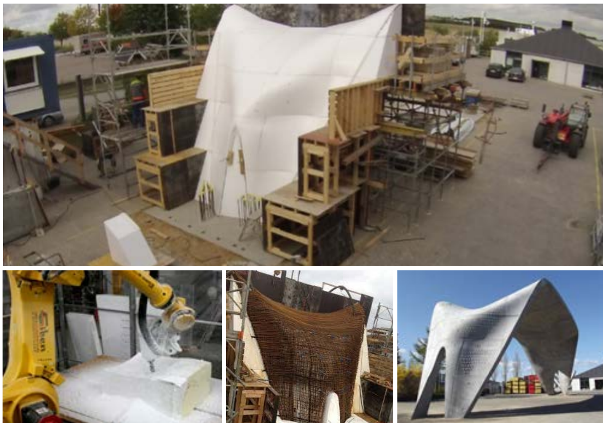
Figure 14: Production process of free-form concrete sculpture using CNC-Milled EPS blocks. source: Tailorcrete
