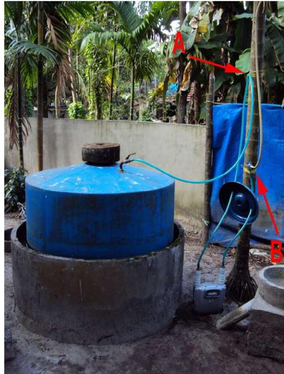
Figure 10 – BIOTECH toilet-linked digester, with fixation point (A) and measurements points (B) of the connected gas meter (Estoppey, 2010, p. 18).
