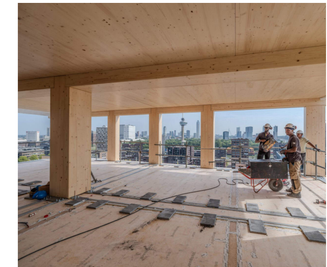
41 - SAWA Rotterdam construction. NICE developments (2025)
