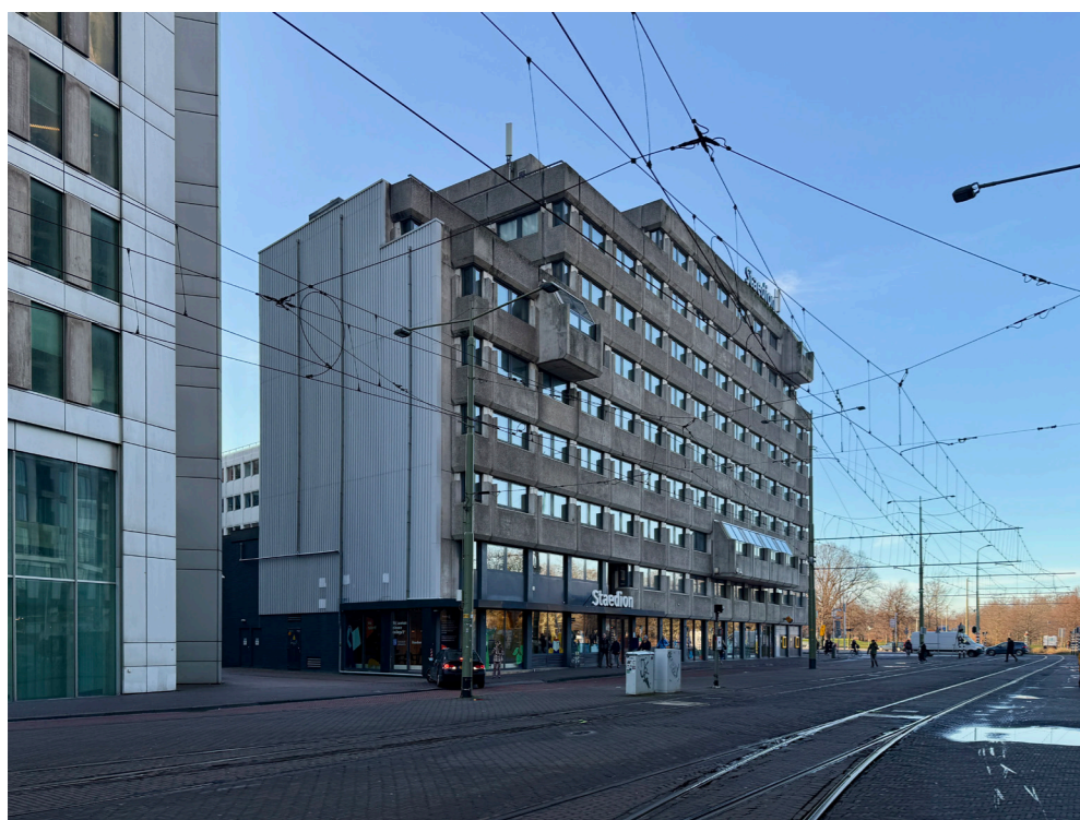
13 (top left) - Example of damage on facade. Own imagery. 14 (bottom left) - Facade with metal sheet cladding. Own imagery. 15 (top right) - Elevation drawing situation 1976. Own imagery. 16 (bottom right) - Elevation drawing situation 2026. Own imagery.
