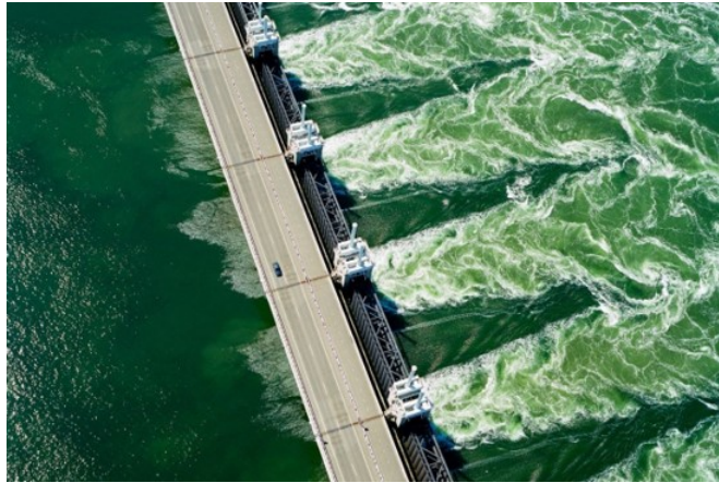
Figure 2.5: Flow structure downstream of the barrier that shows characteristics of grid turbulence (VVV Zeeland, 2018).
